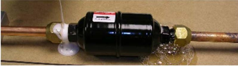
*example of bubbling caused by leakage*
